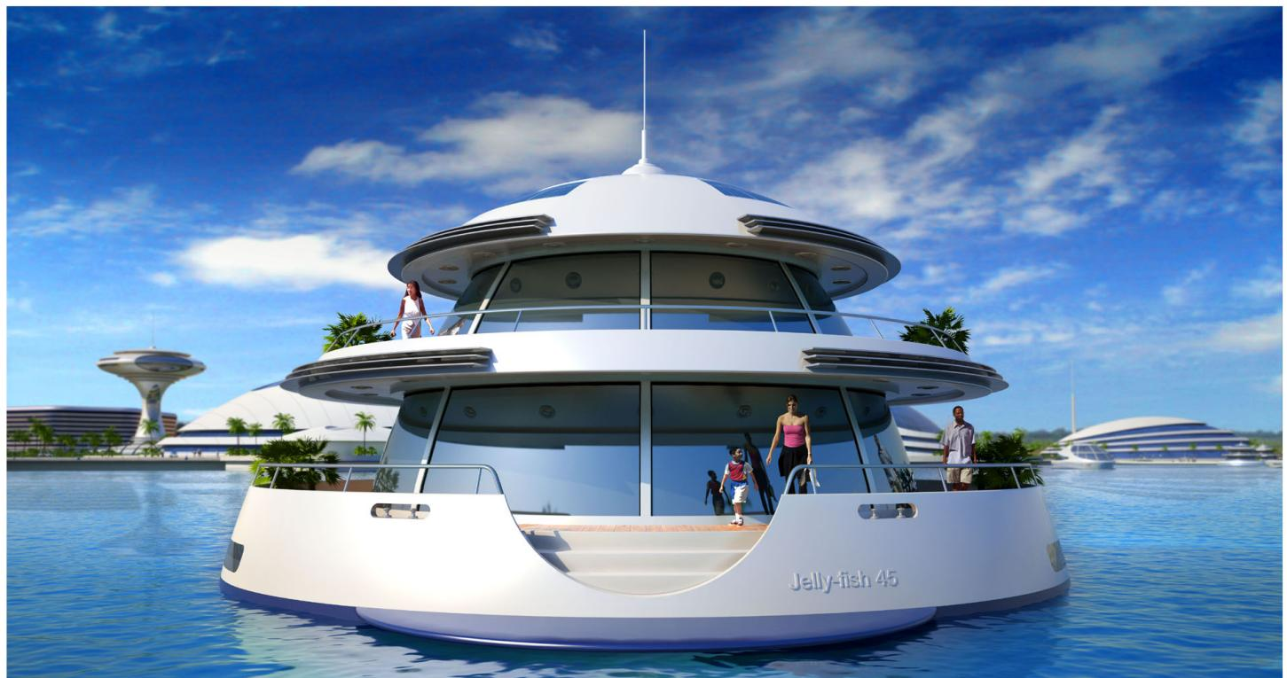
The floating suites are "Jellyfish", structures designed by Zema in 2003. They measure 50 m in diameter and can hold 6/8 beds. The structure is made of aluminium while the bridges are made of teak. The observatory-sphere, which reaches down to a depth of 3 m, is made of how resistant acrylic panels and fitted with a reflective lighting system allowing guests to admire underwater life even at night-time.
